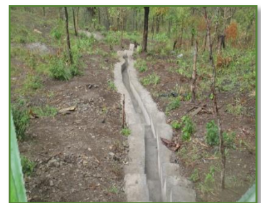
Catch water drain
