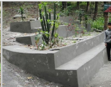
Cement Rubble Masonry wall
