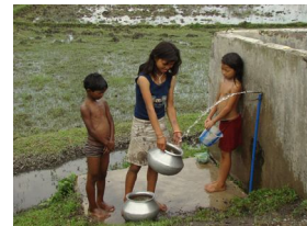
Drinking water facilities
