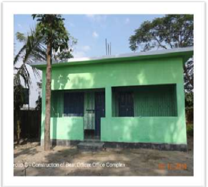
Construction of Beat Office Complex at Jhargram DMU under Gidhni FMU
