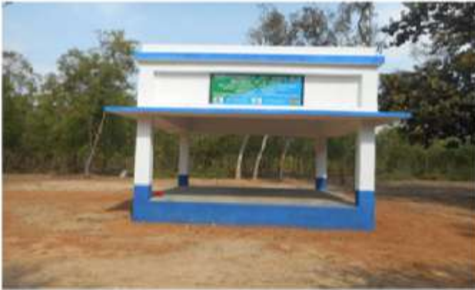
Construction of Atchala at Bankura North DMU under Radhanagar FMU
