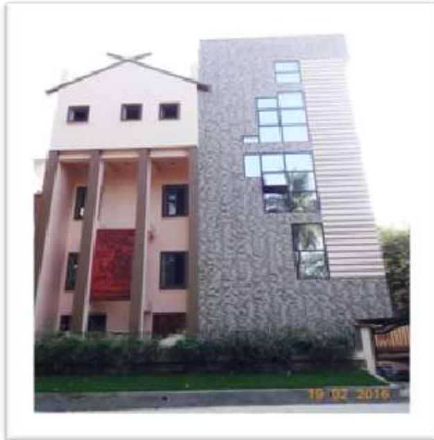
Construction of Bon Bhawan at AE-391, Saltlake City Kolkata
