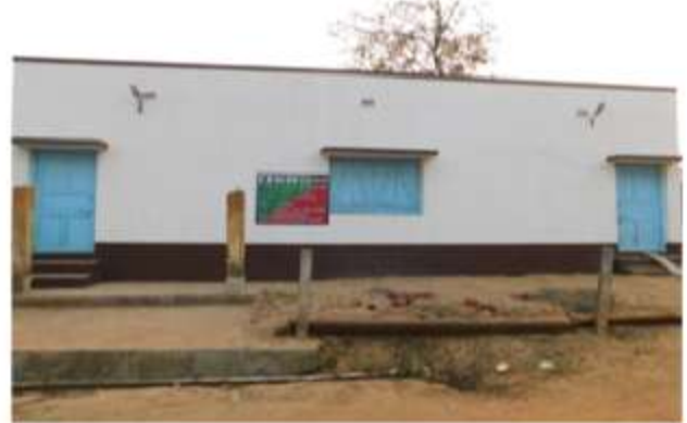
Construction of Community Hall at Bankura North DMU under Beliatore FMU
