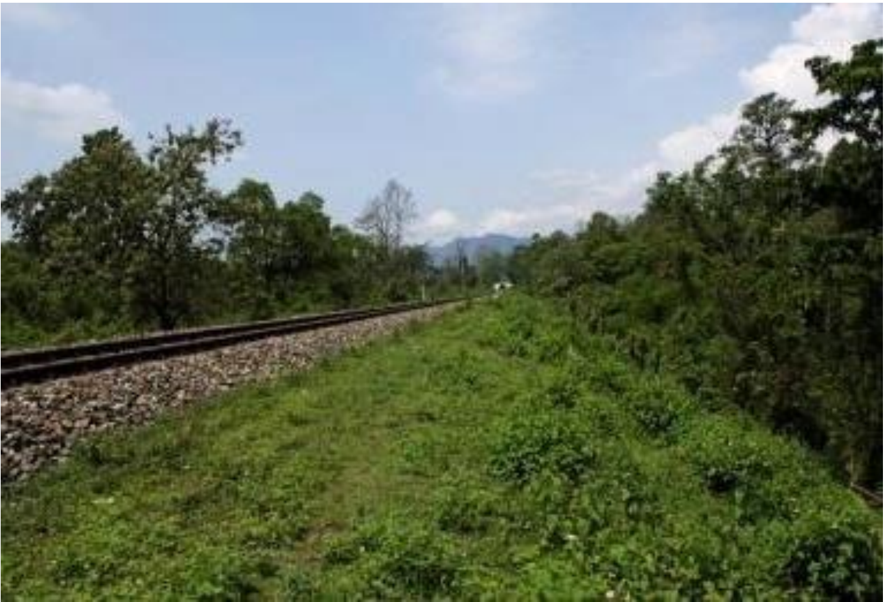
Fig 33: Railway track inside the protected area
